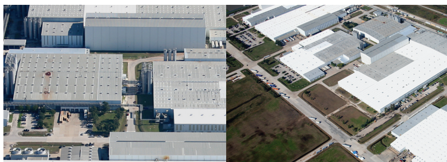
Texas Manufacturing Facility 1 million+ sq. ft. Metal
