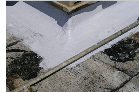
COMPLETELY RE-FLASH AND SEAL ALL SEAMS ON ALL SUBSTRATES
