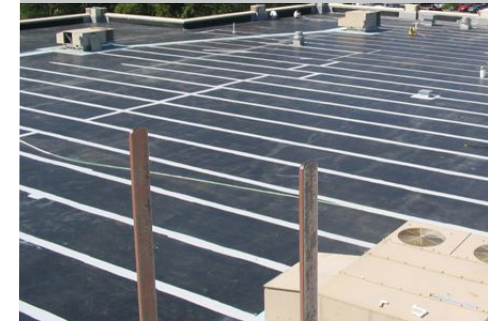
COMPLETELY RE-FLASH AND SEAL ALL SEAMS ON ALL SUBSTRATES
