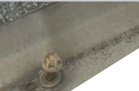
LOOSE FASTENERS
